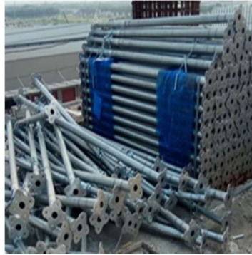
Gambar 2.14 Pipe Support
