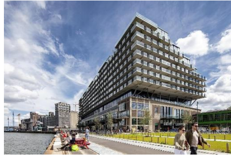
Gambar 2. 3. Fenix I Warehouse Renovation
