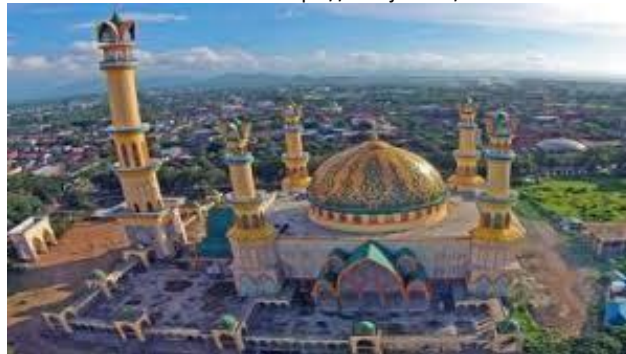
Gambar 8. Tampak Atas Masjid Raya Hubbul Wathan Islamic Center NTB
