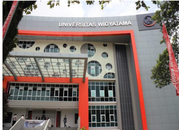
Gambar 1. Fasad Student Center Univ. Widyatama
